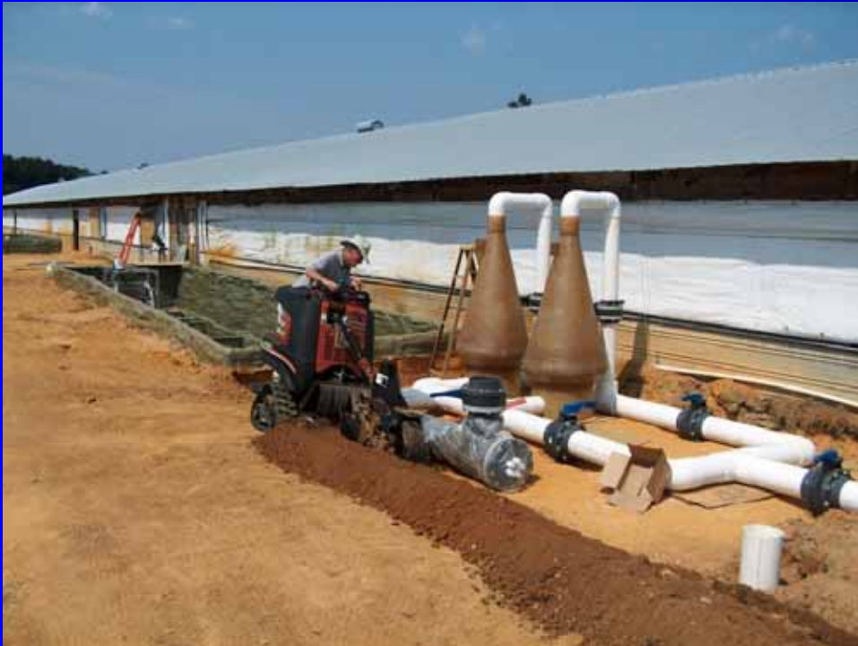
Large Scale Poultry House Conversion, 80% Complete
