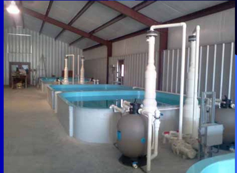
Design / Build of a Staging & Processing Facility
