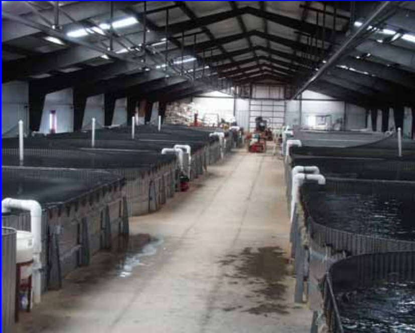
Building 2 Completed (total 32 production Tanks)
